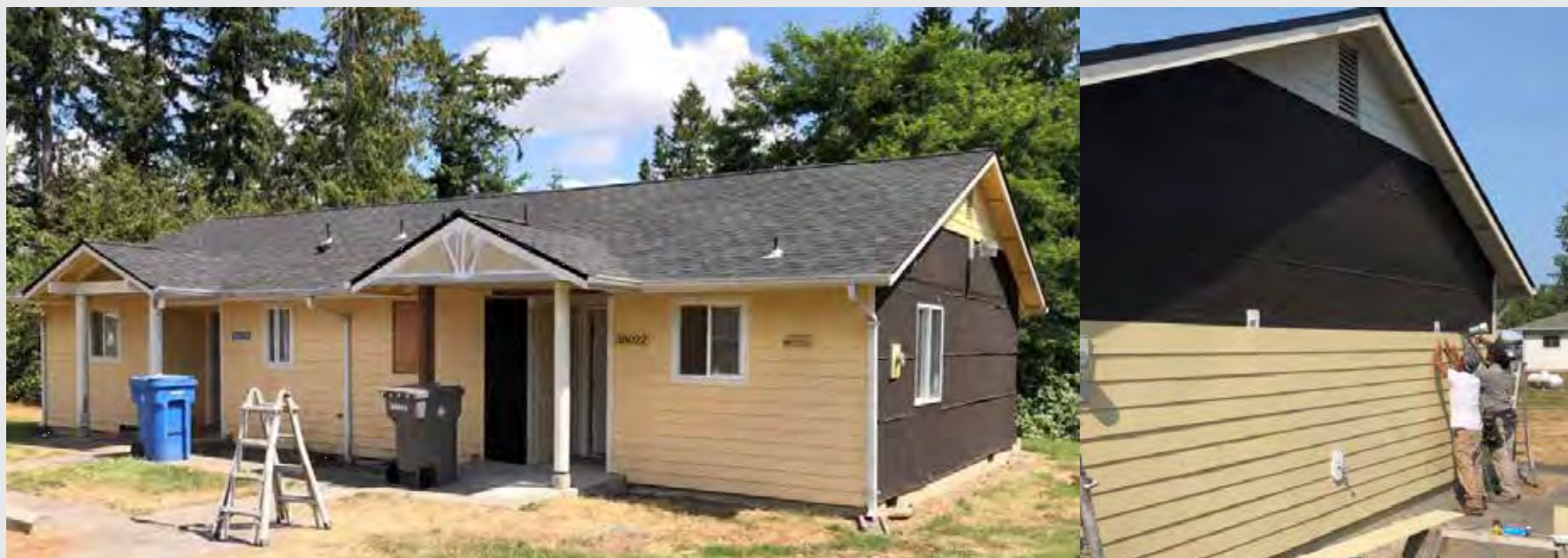
1 Bedroom Duplex - Renovation In Progress - Bathrooms Updated for Accessibility
