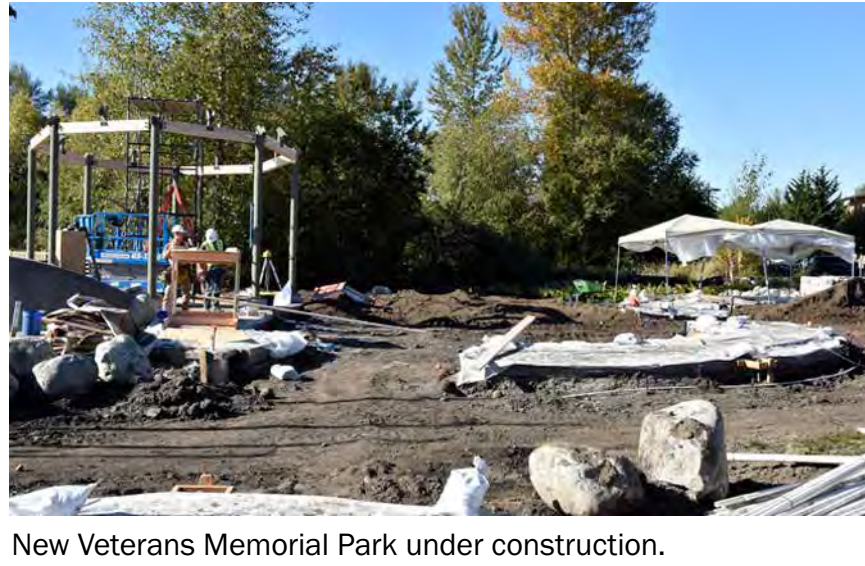
New Veterans Memorial Park under construction.
