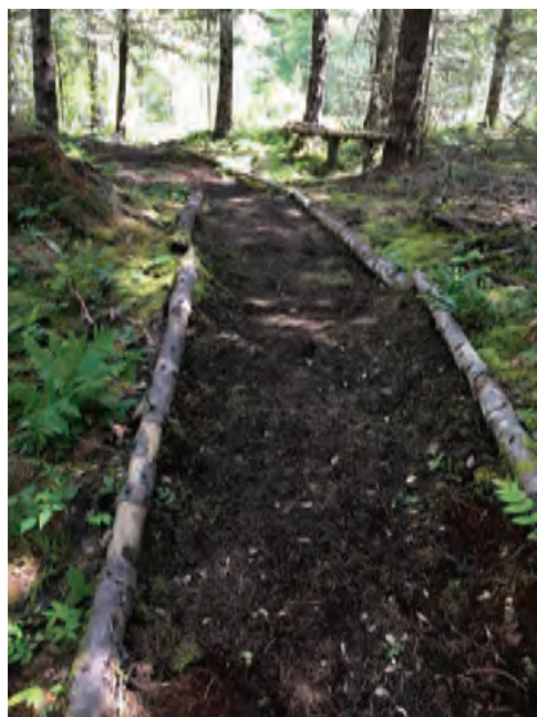
Excellent trail restoration work at Medicine Eagle Flats.
