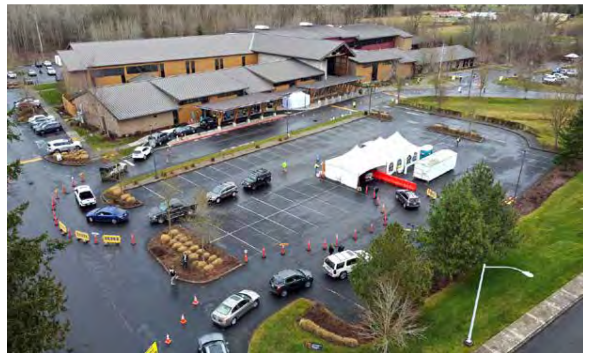
Seen from the air, a panoramic view of the Muckleshoot Health and Wellness Center during its recent COVID-19 vaccination event. Cars lined up by the hundreds on the circular drive around the pow wow grounds waiting to enter the white intake tent before receiving their vaccine at friendly and efficient drive-through stations in front of the building. At right in the background is the monitoring area where participants waited for 15 minutes before continuing their day. (Ken Lambert / The Seattle Times)
