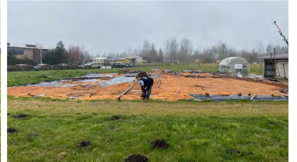
The remodel begins.
