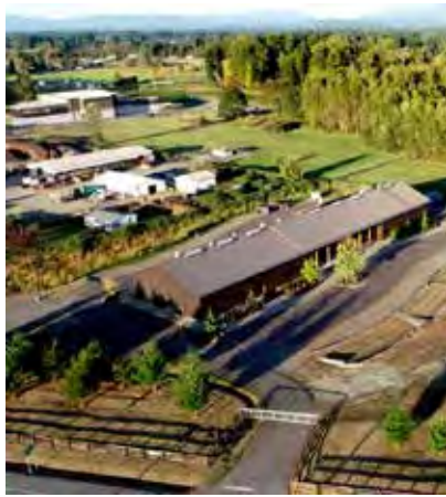
Elk House with Public Works in background
