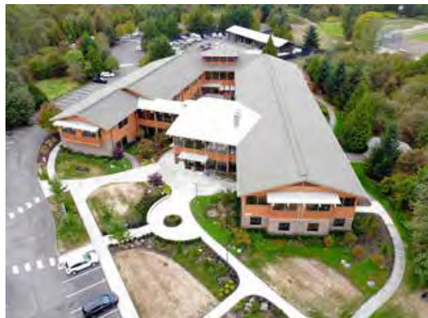
Muckleshoot Tribal Headquarters, the Philip Starr Building
