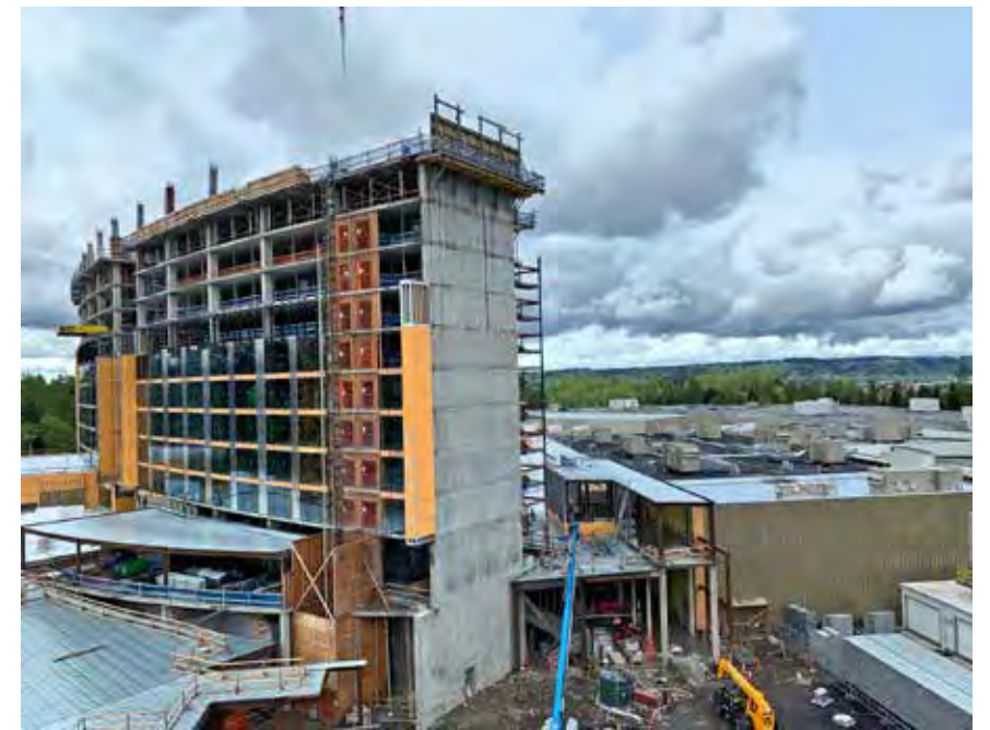
The new hotel has topped out.
