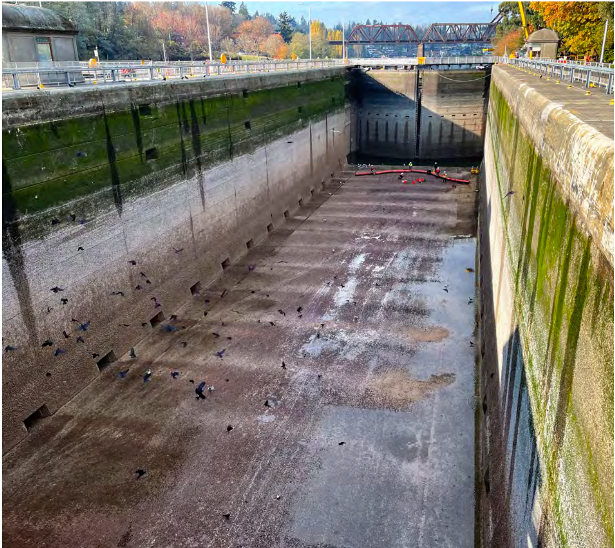
This is a picture of the Ballard large lockage empty of water for their annual cleaning.
