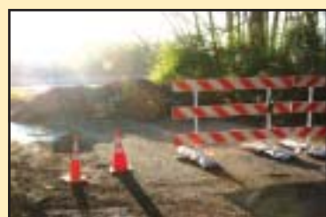
New berm and signage at road's end
